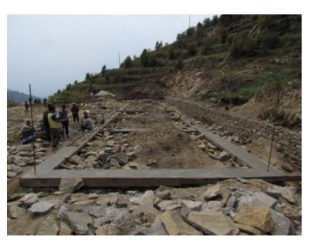
They have not collected inadequate gravel (Crash stone). Only half of the total gravel is seen at the site, but they are going to supply the rest of the gravel as they need it quite soon for RCC.
