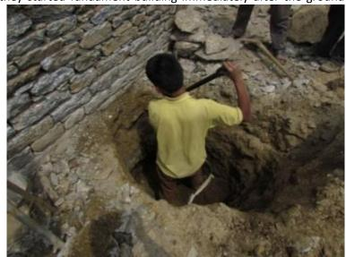
I let constructors dig out 6 different places with random sample and took measurement and photographs of the fundament. I found all measurement and quality construction to a satisfactory level.
